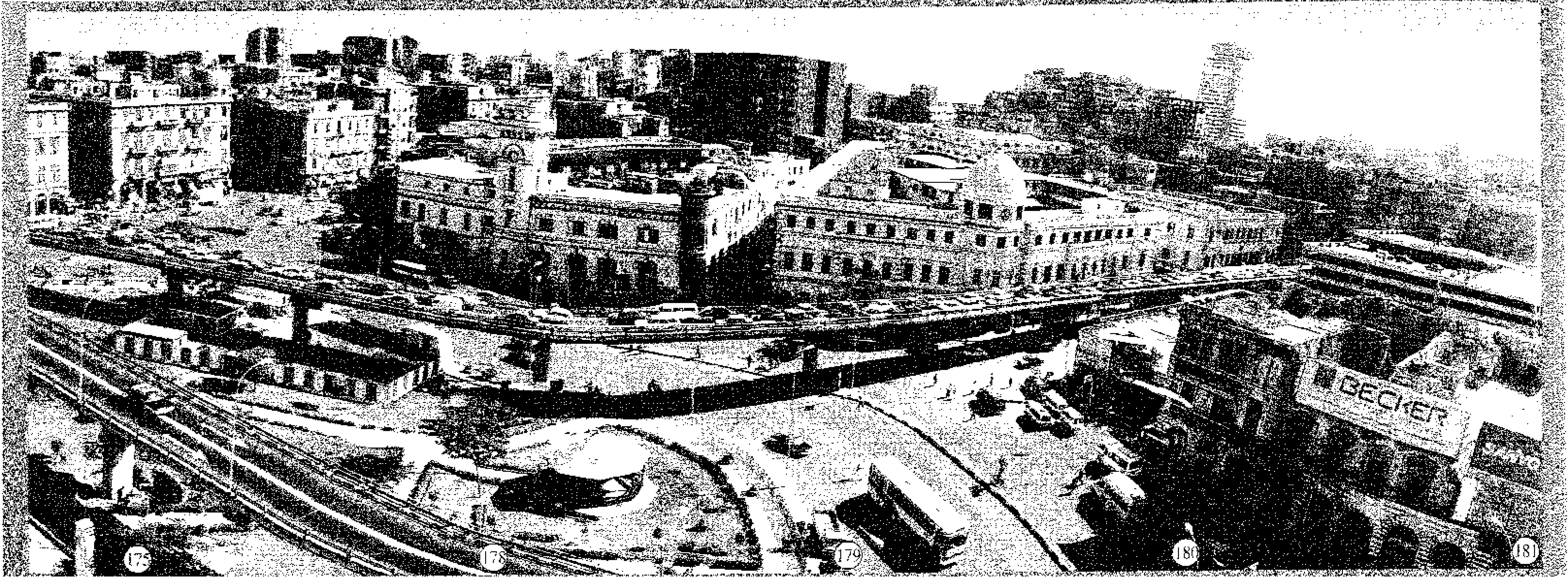
A Group of Historical / Architectural Valuable Buildings shaping together an Urban & Heritage Panorama. "Matatiya Complex Building" (181) & "Mudiriyat El-Shuun El-Sihiya" (180) & "Postoffice Building" (179) & "Matatiq El-Qahira" (178) , "Funduq El-Ataba" or "Parlament Hotel" (175)
